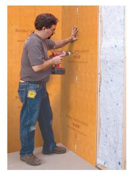
the case of stud framing, KERDI-BOARD is attached with screws and washers from the matching hardware system.
